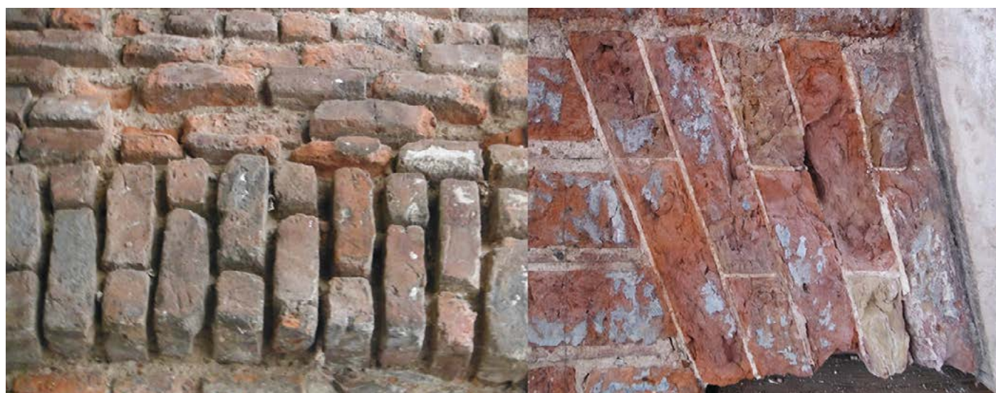
Figure 3 Comparison of the fabric of the window heads in the back wall (left) and the façade (right). Photographs by Sara Pavia.
