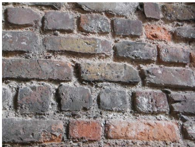
Figure 5 Detail of the brick bond in the back wall. Photograph by Sara Pavia.
